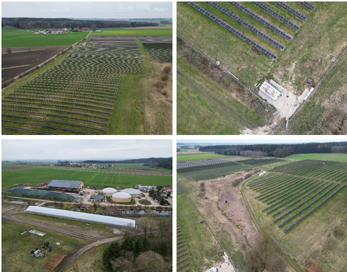
Figure 1: Aerial view of the Maierhof PV installation in Buttenwiesen (near Augsburg, Germany), captured via drone during the on-site inspection (24 March 2024) to assess optimal placement of measurement and monitoring equipment.
