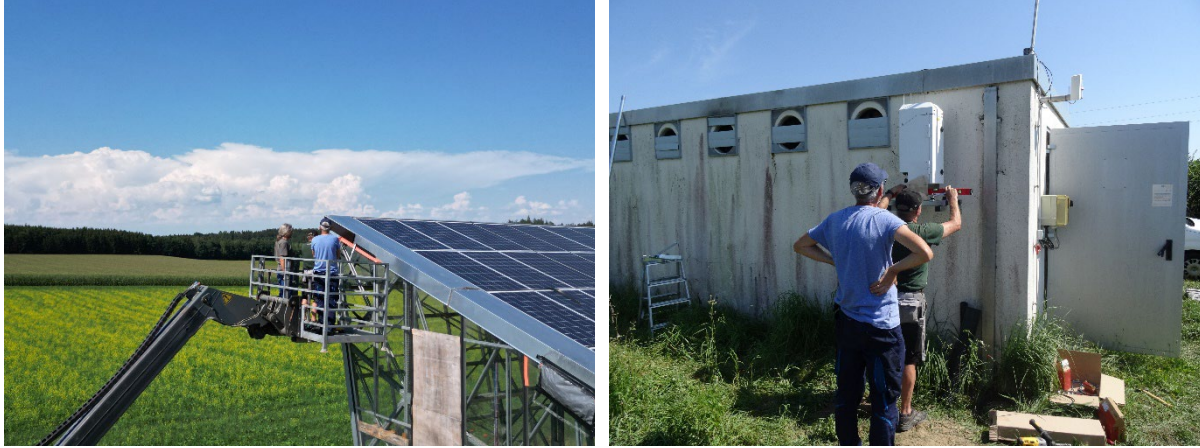
Figure 8: Photos of the installation work, on the left the camera installation in Illemad using a telehandler, on the right the installation of the SkyVue8 on the exterior wall of the technical building.
