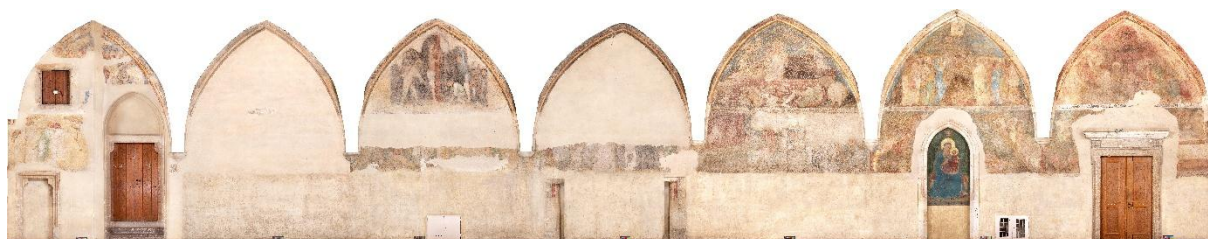
Figure 7: Photogrammetric image of the East walk of the cloister. © Jiří Vidman, Pavel Hlavenka.
