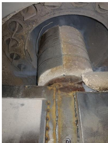
Figure 4.16 Clay insert mounted above the grate
