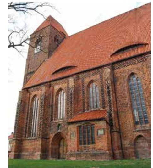
Figure 1: St. Johannes church in Werben, southwestern part with steeple
