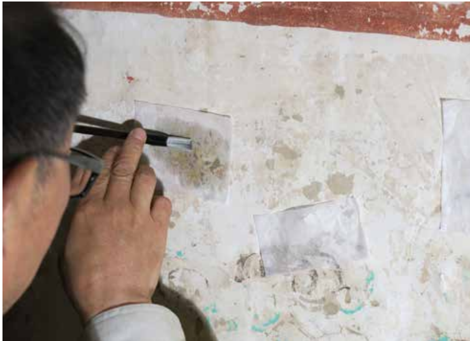
Figure 8: Relaying of exfoliated areas was undertaken with water and water: ethanol mixes applied with brushes through paper tissue.
