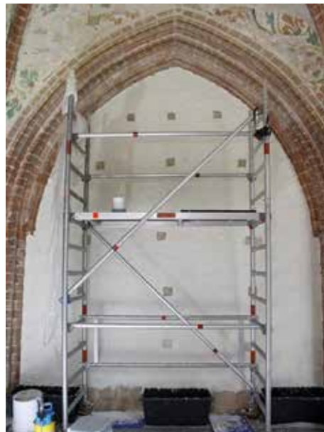
Figure 2: Application of desalination poultices
