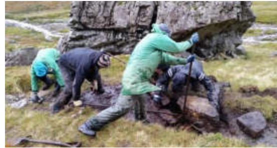
Building drainage ditch on Ben Nevis trail
