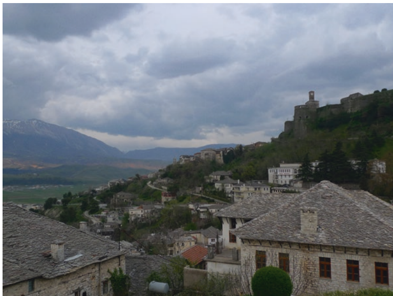
Fig. 2 Roof landscape with traditional stone cover in Gjirokastra, Albania (Source: M. Ripp)
