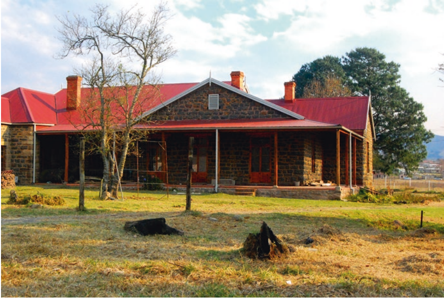
Fig. 2 Montrose House shortly after most of the repair work had been completed. See Mpophomeni in the background (Photo: Kelly Goss 2013)
