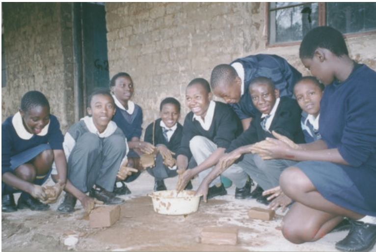
Fig. 1 Children making mud bricks for plugging cracks in walls (Photo: Genna Nashem 2002)
