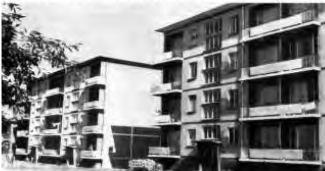
Sofia. Residential building from the first large-panel system building residential complex "Tolstoy", 1960. Plan and view at its completion Project of "NISI", eng. Georgi Brankov and team, architects are D. Davidov and K. Panayotov
