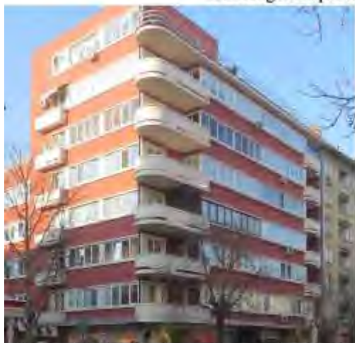
Sofia, 48, Vitosha Blvd. Building cooperative, 1937-1938, arch. Radoslav Radoslavov and arch. Konstantin Djangozov.
