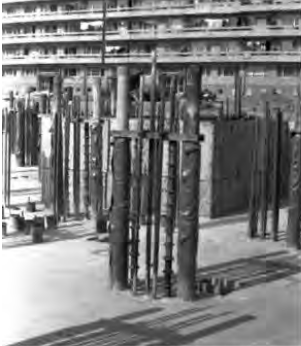
Mounting installation for the the Lift-Slab Method of construction
