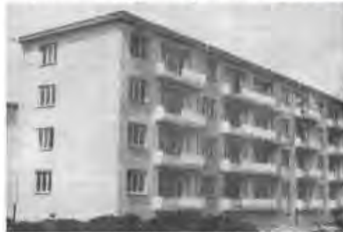
Sofia. Residential building from the first large-panel system building residential complex "Tolstoy", 1960. Plan and view at its completion Project of "NISI", eng. Georgi Brankov and team, architects are D. Davidov and K. Panayotov
