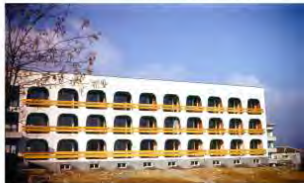
Sofia, Apartment block. Monolithic on-site cast concrete structure, 1980's
