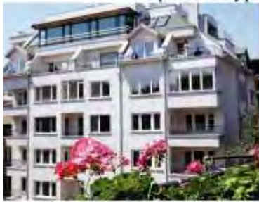
Sofia, "Trakia" str, 1996. Building with two attic floors
