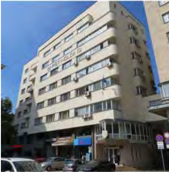
Sofia, 3 "Moskovska" Str. Corner with "Malko Tarnovo" Str. Building cooperative "Karadzhatia", 1928-1929, arch. Krastan Gechev and arch. Peter Karasimeonov.
