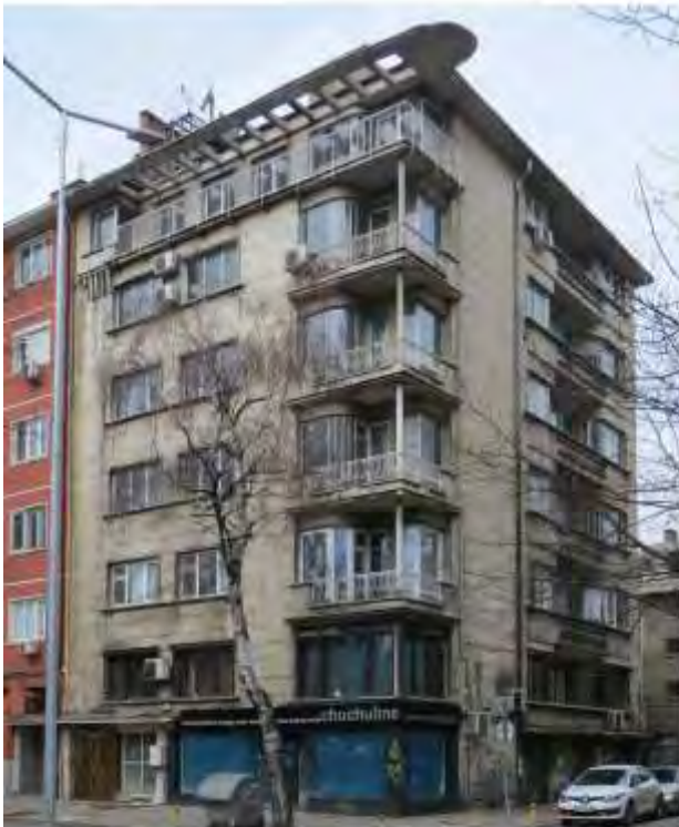
Sofia, the corner of "Evl. And Hr. Georgievi" Blvd. and "Geneva" Str. Building Cooperative, 1943, design by arch. Vasko Vasilev.
