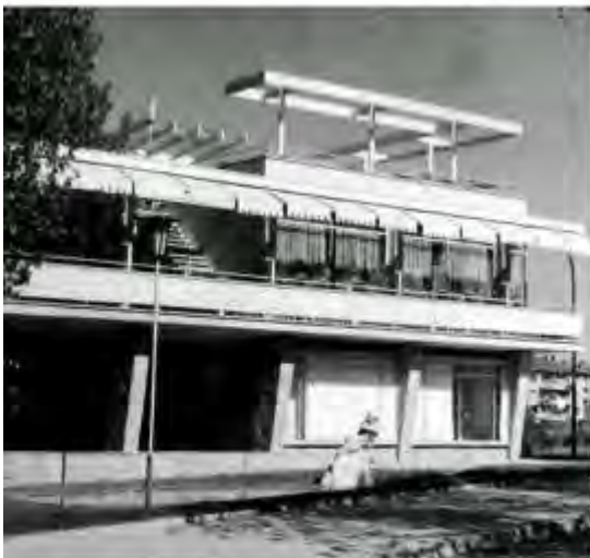
Sofia. Residential complex "Yavorov", coffee shop "The fairy", design by Arch. Vasil Valchanov
