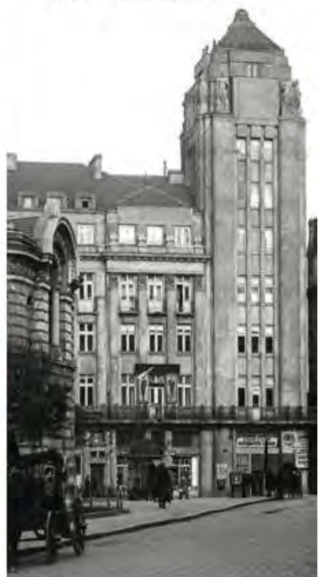
Sofia, the corner of "Serdika" Str. and "Triaditsa" Str. "Musala" building cooperative, 1925, Arch. Kosta Nikolov
