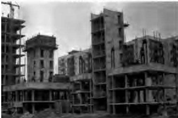
Mounting installation for the the Lift-Slab Method of construction
