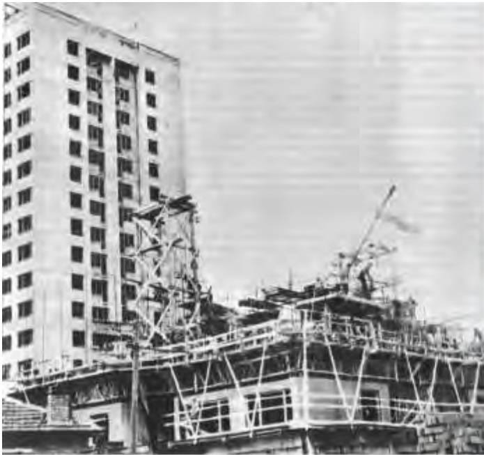
Sofia, apartment blocks (one under construction). First use of slipform construction, 1966
