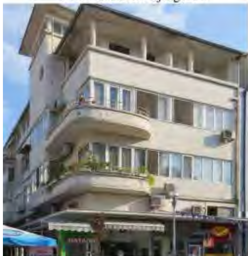
Varna, 1 Knyaz Boris I Blvd. Building cooperative, 1938, Arch. Stefan Venedik Popov
