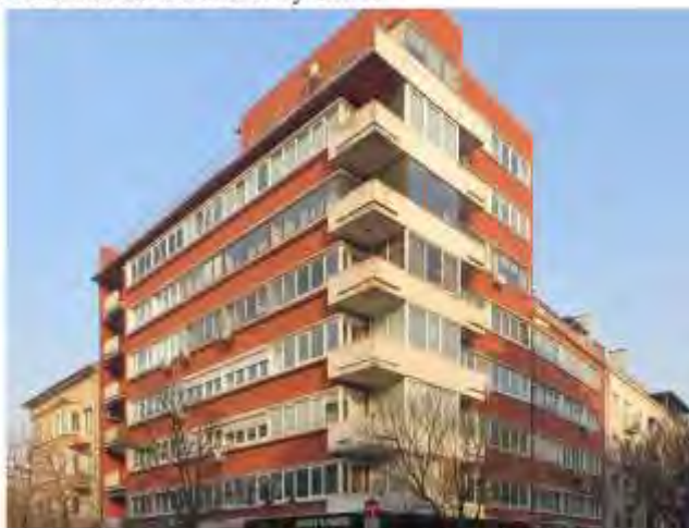
Sofia, 59, Vitosha Blvd. Building cooperative, 1938-1939, Arch. Radoslav Radoslavov and arch. Konstantin Djangozov.
