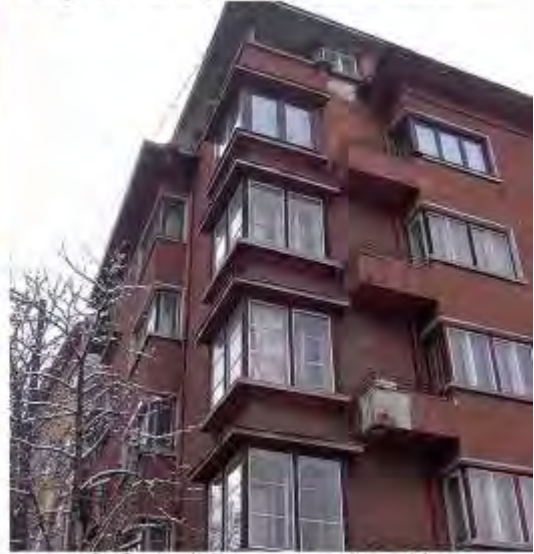
Sofia. Building cooperative with a constructivist vision, 1934.
