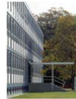
Bunde Eisenmann Bau Andy Warhol Building Offenbach
