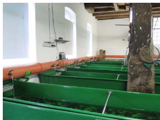
Abb. 7: Wasserversorgung der Langstrombecken (K.Detloff).
