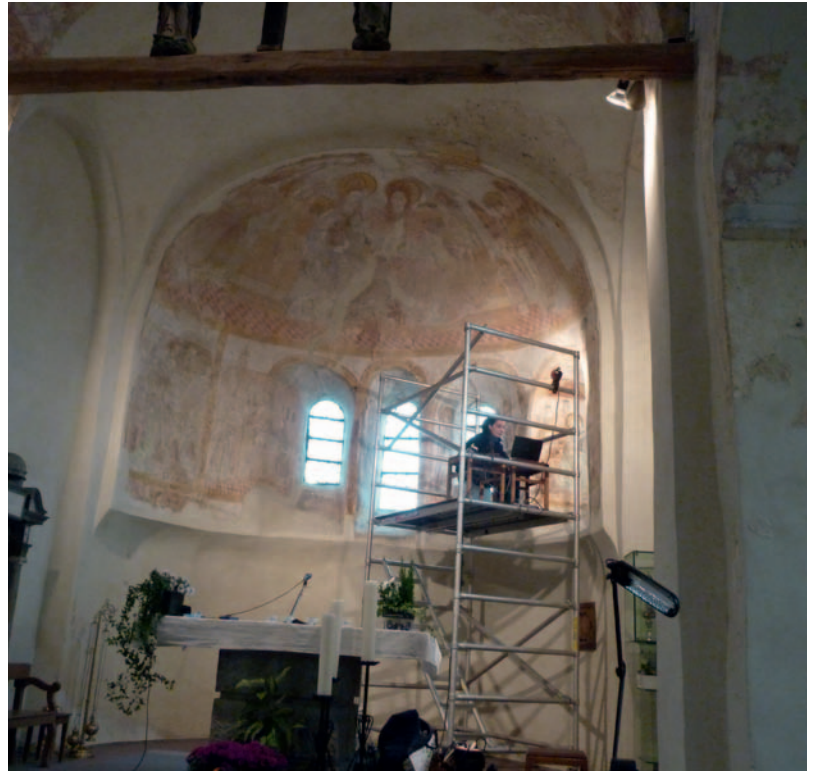
Fig. 13: Bois, Saint Lambert's Church, choir. Work on site by Estelle De Groote (Foto I. Hans-Collas, 2012).
