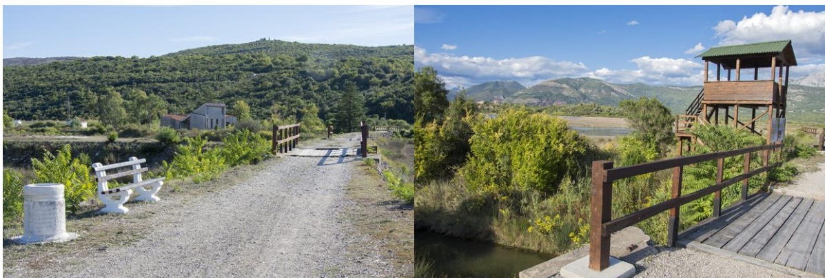
Figure 20: More newly constructed benches and litter bins (left), as well as renovated bridges and a new observation tower with information boards (right) complement the touristic infrastructure in Tivat salina (photos: CZIP)
