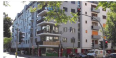
Photo 1: Multi-story passive house at Amimplatz, Berlin-Prezler Berg built for 123 persons (41 dwellings) and covering an area of 4,900 \text{m}^2 .
