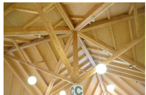
Abb. 160: Detail Strebenbündel [52]
