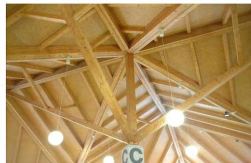
Abb. 160: Detail Strebenbündel [52]
