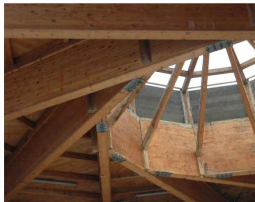
Abb. 232: Detail Trägeranschlüsse [52]
