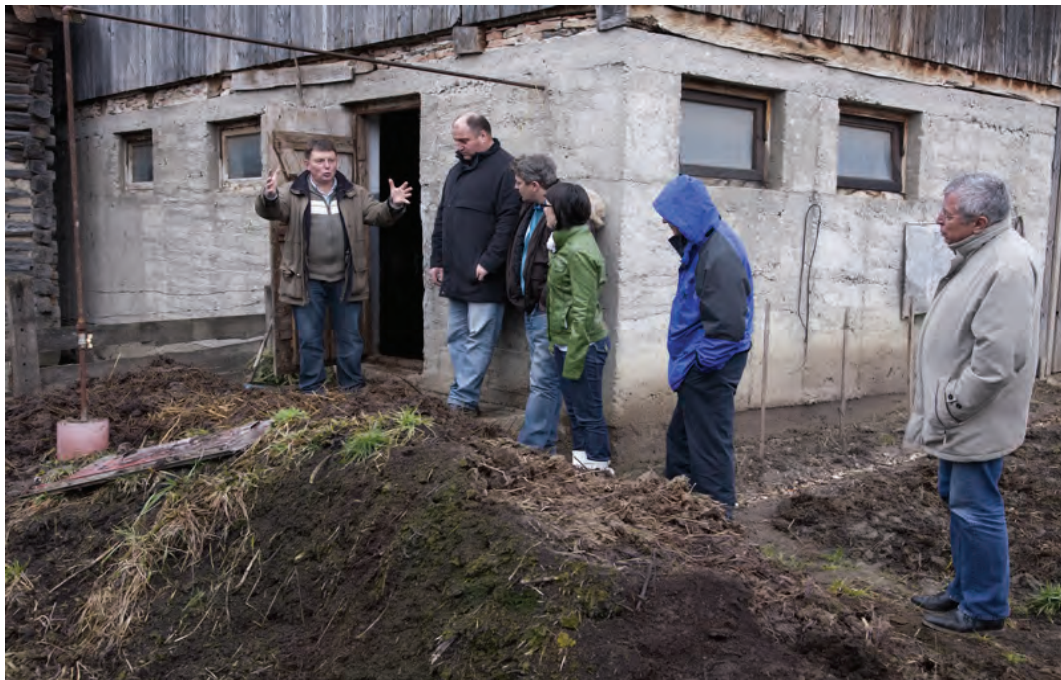
Figure 13: Kálmán Sándor (left) explains his small scale biogas unit on a dung pile (see gas collecting vessel on the left side and gas main to the kitchen)
