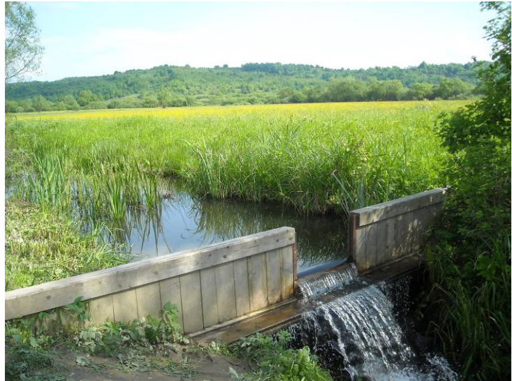
Figure 40: Melioration channel in the Narcissi Valley.
