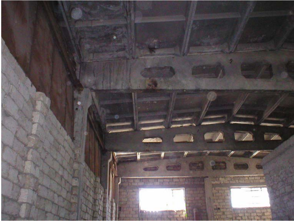
Exhibit 11 Training Center, Large Hall
