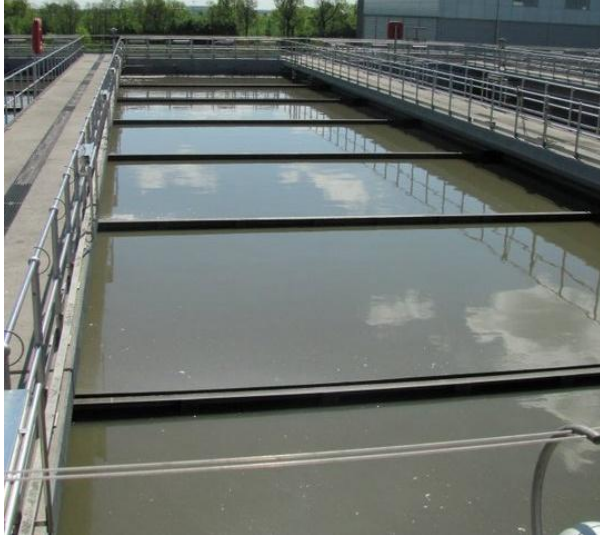
FIGURE 7: PRIMARY SEDIMENTATION TANK
