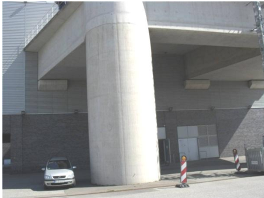
FIGURE 4: INLET STRUCTURE, COLUMNS ARE HOLLOW AND TRANSPORT THE WASTEWATER
