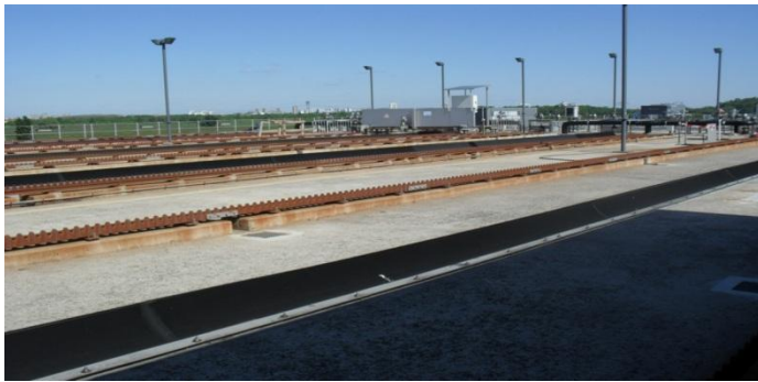
FIGURE 6: GRIT CHAMBER, COVERED
