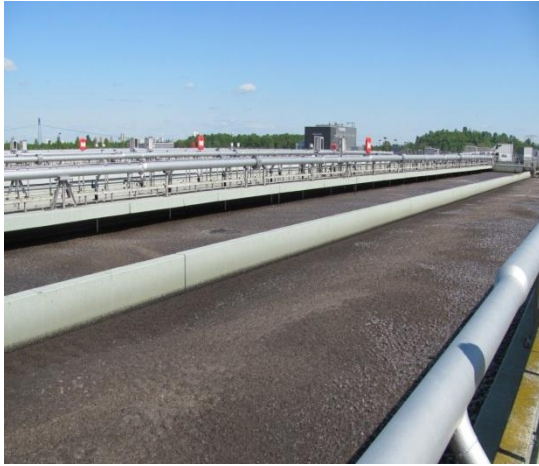
FIGURE 9: AEROBIC ZONE OF BIOLOGICAL TREATMENT
