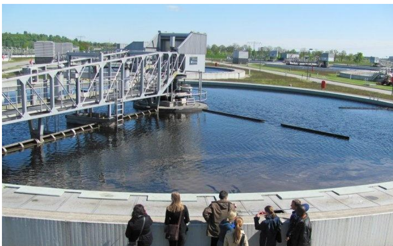
FIGURE 11: SECONDARY SEDIMENTATION TANK
