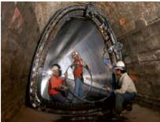
Picture 2. Physical evaluation of sewer systems
