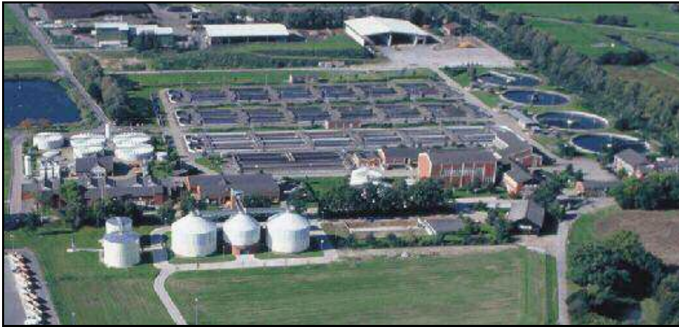
Figure 5. Wastewater Treatment Plant Braunschweig
