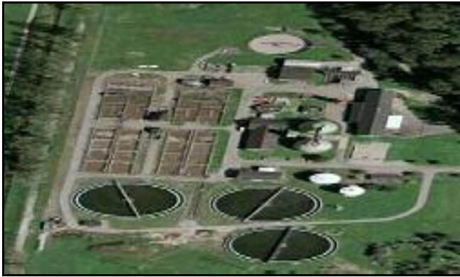
Figure 6. Wastewater Treatment Plant Baden Baden Sinzheim
