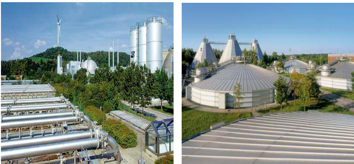
Photograph 1: (Left) -Wastewater Treatment Plant Gut Großlappen;
