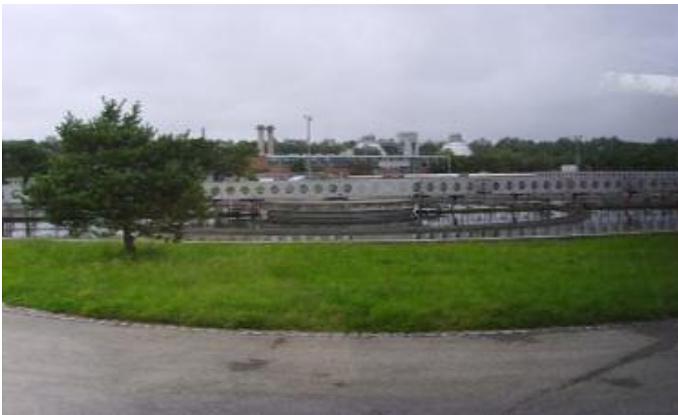
Photograph 5: Primary sedimentation tank
