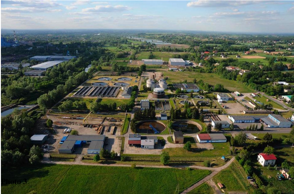
Figure 3. Wastewater treatment plant in Komorowice
